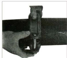
Housing installation
